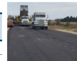
Figure 1. Placement of nonwoven geotextile layer
