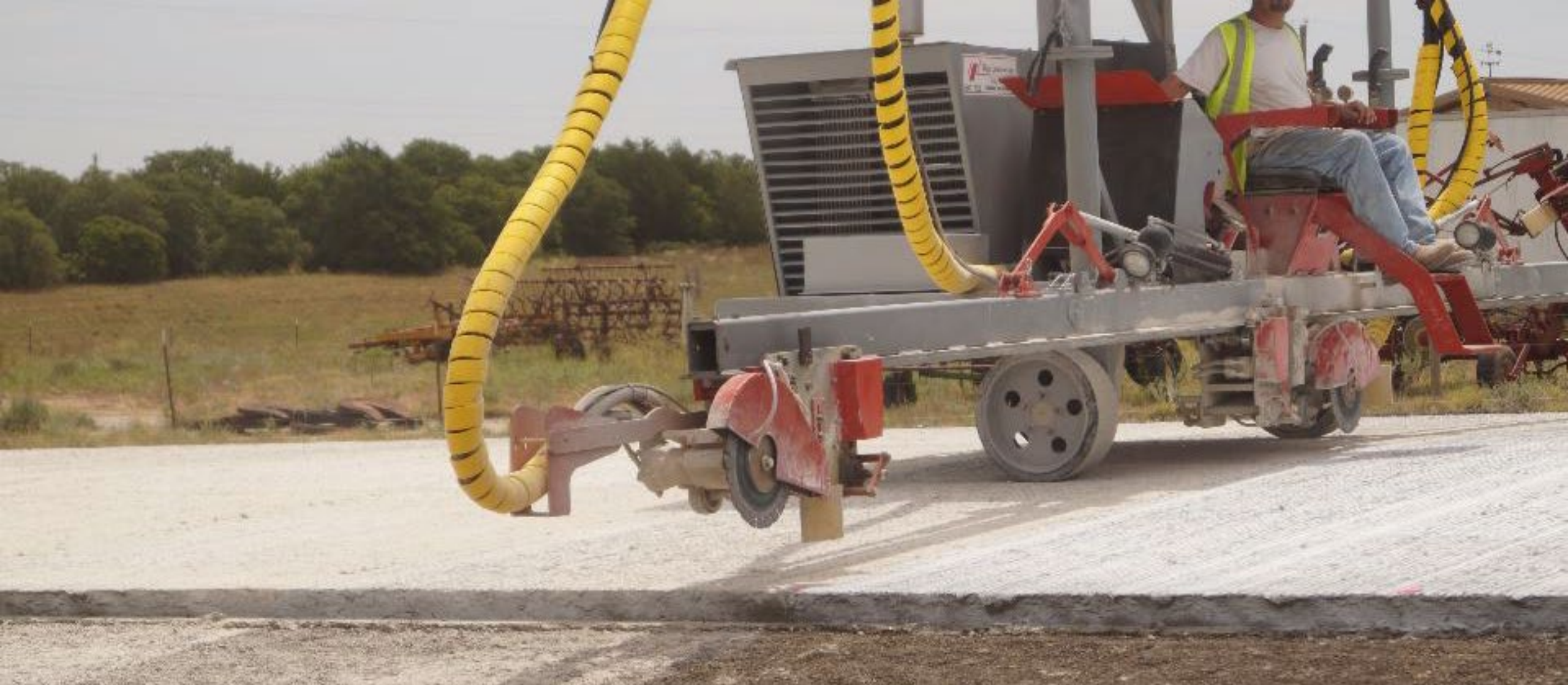
Closeup of Span Saw
