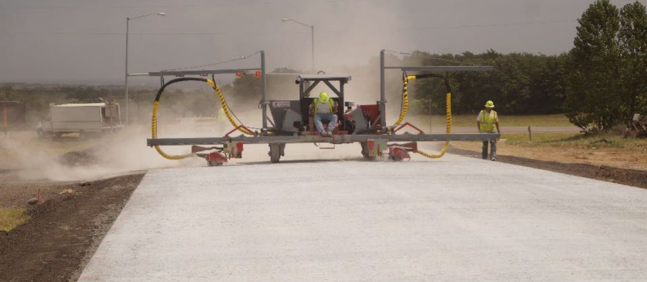
Span Saw Cutting Transverse Joints
